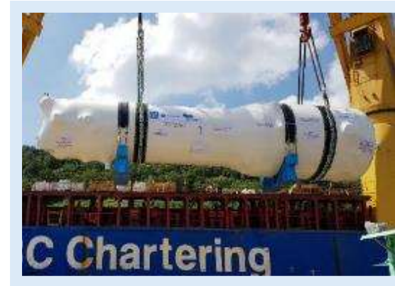
Watts Bar #1,2 Steam Generators
