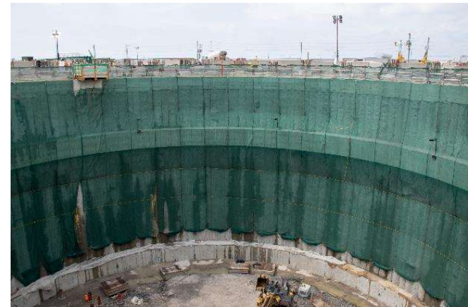
Reactor building shaft excavation
