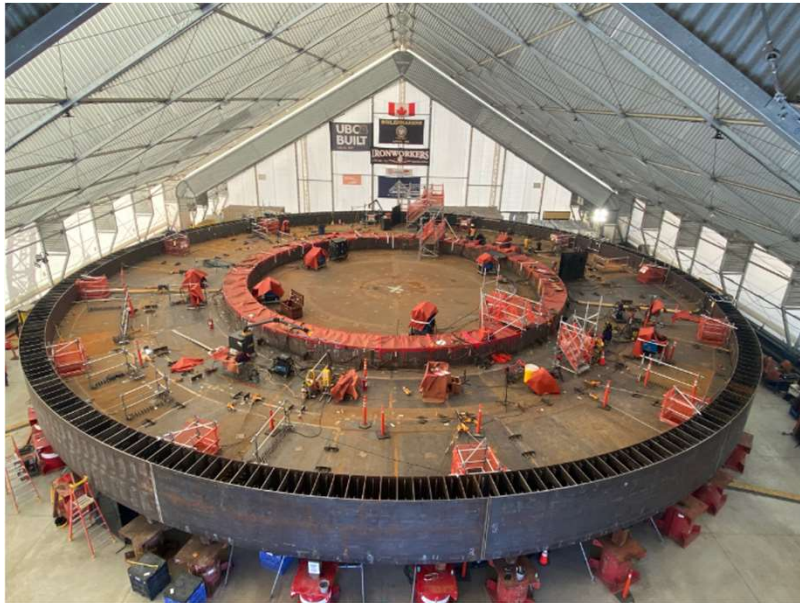
Reactor Building Basemat
