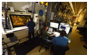
Hot Fuel Examination Facility
