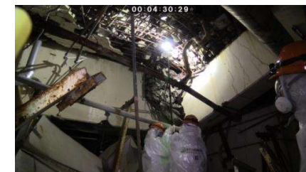
Unit 3 investigations Figure source NRA
