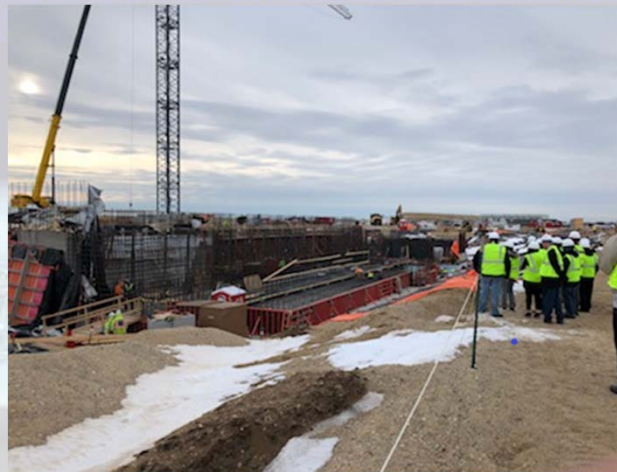
SHINE Construction Site (February 2020)
